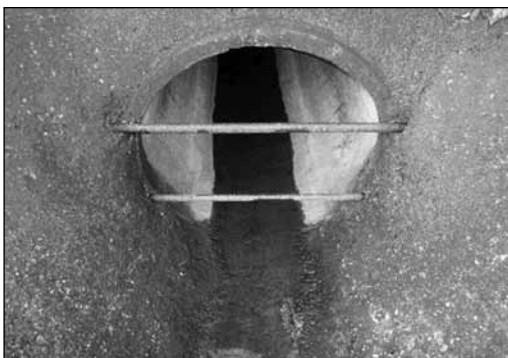
Outfall # 8, the furthest north, flows east directly into the Scugog River.
