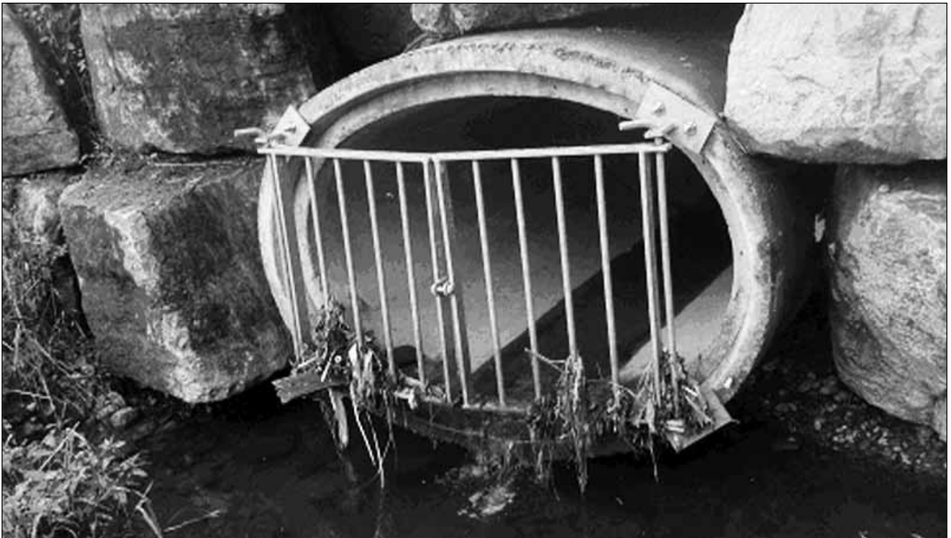
Storm sewer outfall in Lindsay on the Scugog River
