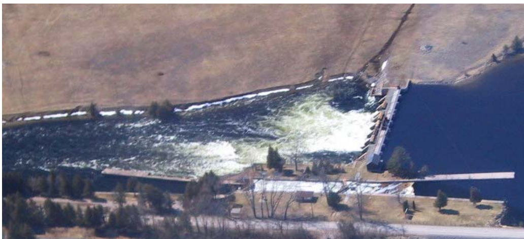
Sawyer Creek Dam - Otonabee River south of Lakefield
