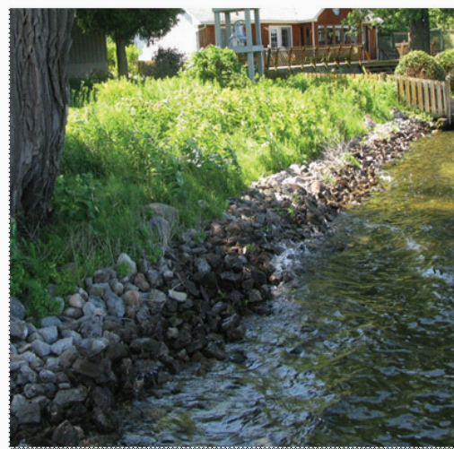
Fig. 3 (After): Sloped rock and natural vegetation provide a healthy and stable shoreline.
